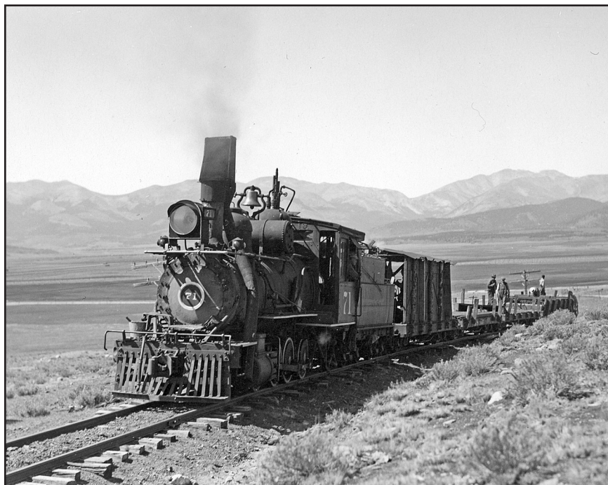
Colorado & Southern 71, with the dismantling train on Kenosha Pass, at the northern edge of South Park on September 18, 1938. – R. H. Kindig photo.
